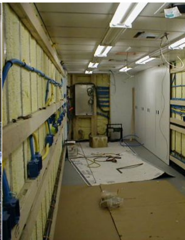
What was left of MdBioLab's two forward air conditioners after a visit with a short bridge
